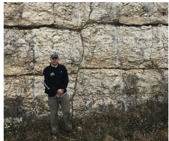
Ross Ledoux investigating hybrid shear fractures in the Buda Limestone, West Texas.
